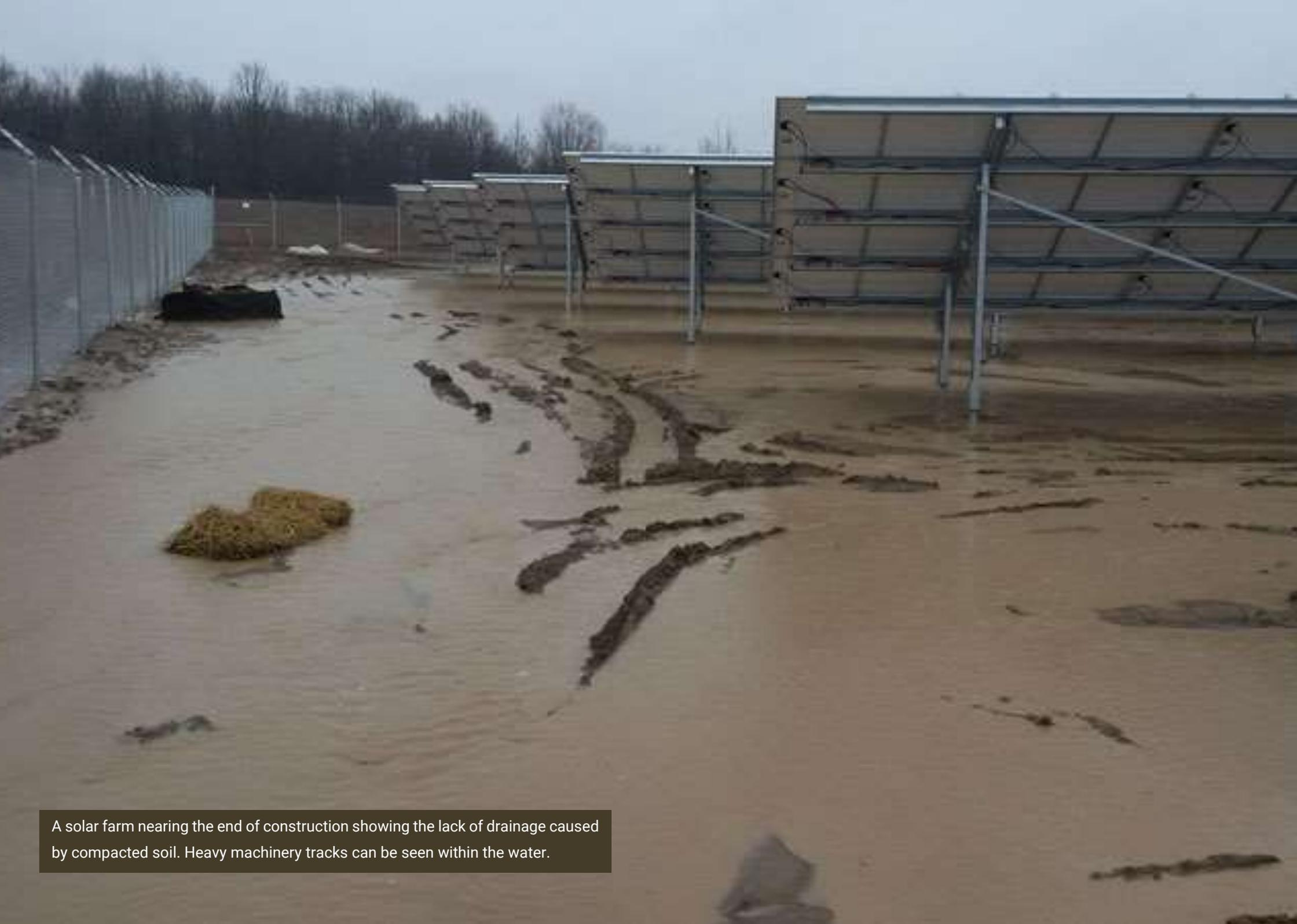
A solar farm nearing the end of construction showing the lack of drainage caused by compacted soil. Heavy machinery tracks can be seen within the water.
