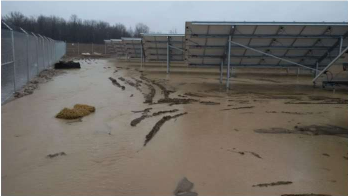
Fig.X+1 - Typical standing surface water present following soil compaction during typical solar farm construction
